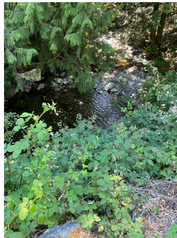
W4. Looking at pool from top of culvert
